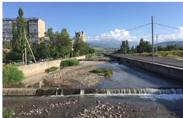
Figure 7: Concrete banks and dissipation walls along the rivers (drawings and photo by the authors)
